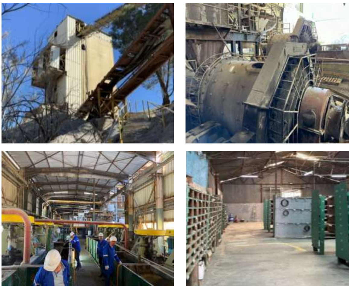
Figure 10 SAMINE Facilities Photographs (pre-con tower, mill, flotation, stores)
